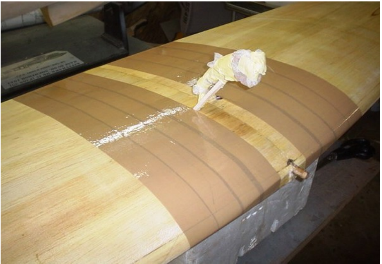
3). Tape top of wing to ensure bog wont stick and then fit wing, bog squeezes out of joint and meets bog applied over rough planking.
